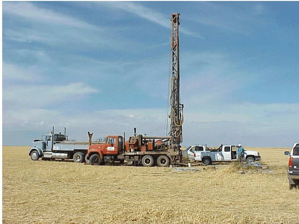
Dollman's Water Well Drilling - Rig Set Up Over Unused Well
