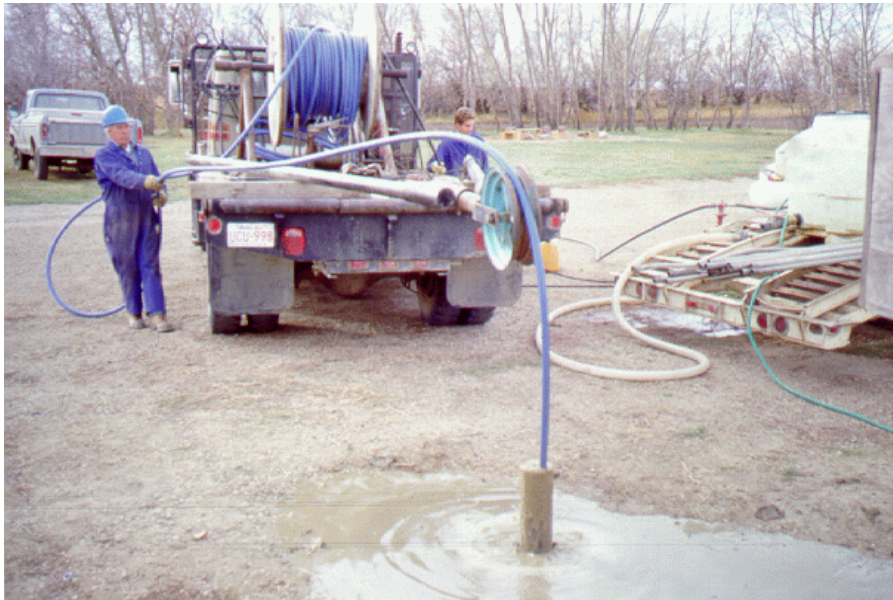
Lifewater Drilling Cementing Unused Well
