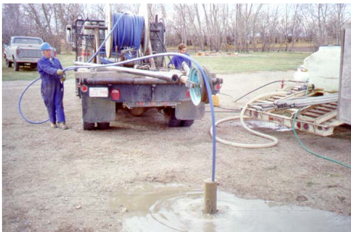
Lifewater Drilling Grouting Unused Well near Wrentham, AB
